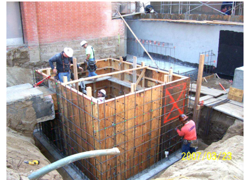
Forming West Side Vault Walls
