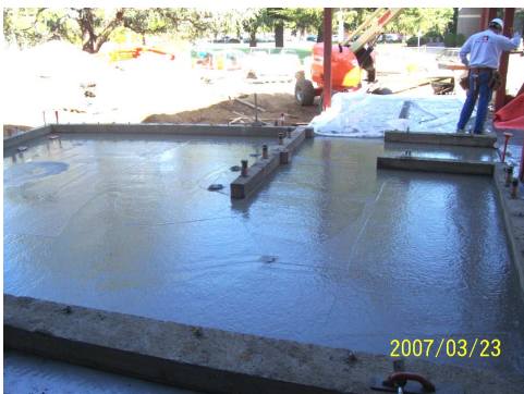
Finishing North Side Slab-on-Grade
