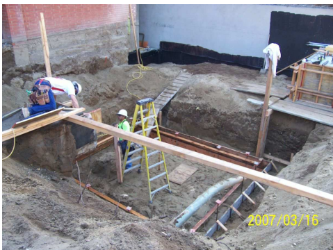
Working on Vault & Steam Tunnel
