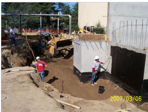
West Side Waterproofing and Backfill
