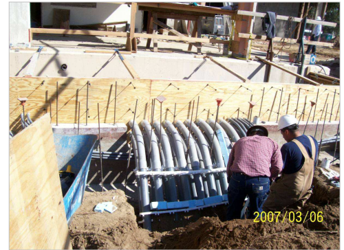
Conduits From Basement Electrical Room
