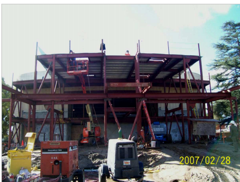
Roof Decking at North Side Addition
