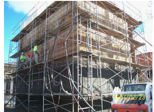
Shotcreting SW Corner Shear Wall
