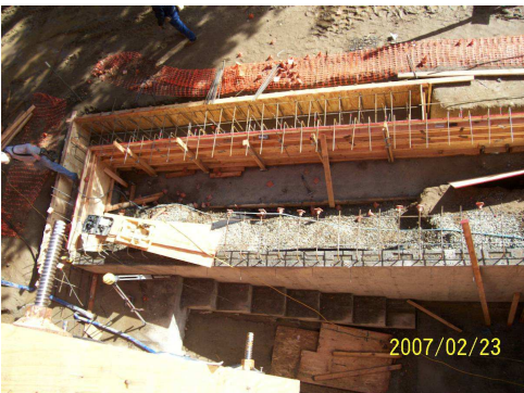
Stem Wall Forms Around East Side Stairs
