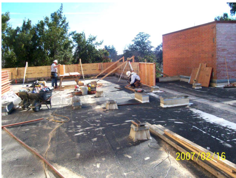
Erecting Parapet Forms at South Building
