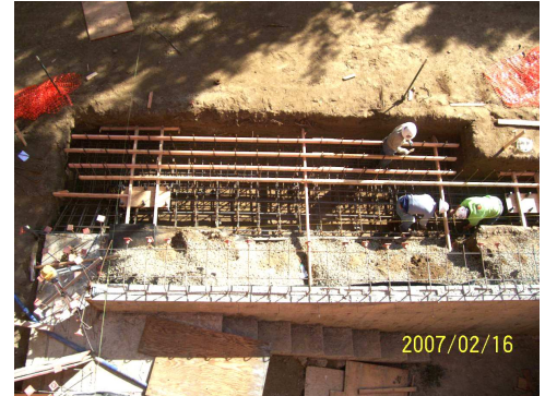
Installing Rebar at East Side Footing
