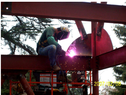
Welding Connection at North Side Steel
