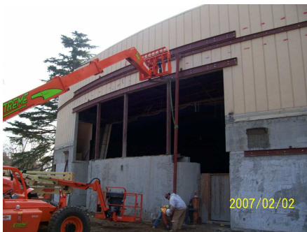
North Side Steel Channels Bolted Building
