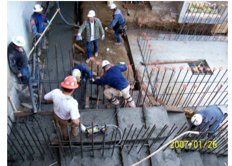
Pouring West Side Elevator/Stairs Footing
