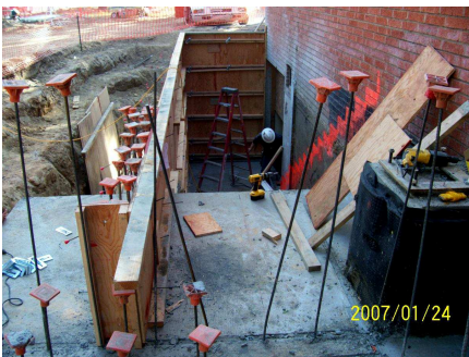
East Side Stairs Wall Formwork
