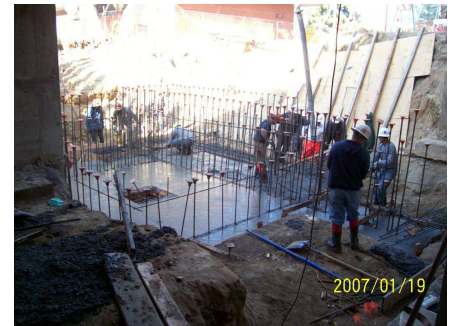
Pouring West Side Elevator/Stairs Footing
