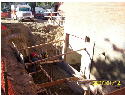
Installing Rebar for East Side Stairs
