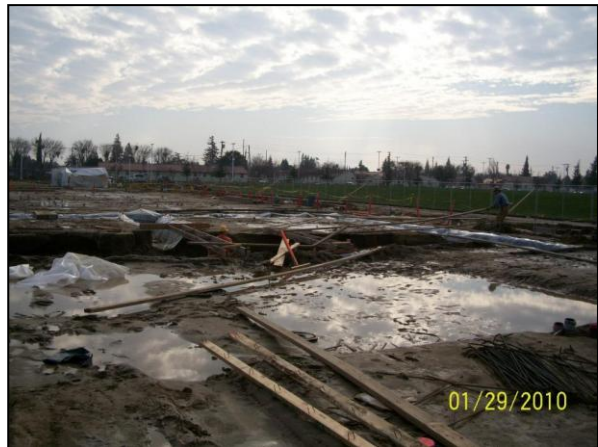
Removing Visqueen from Slab
