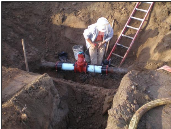
Installing Additional Water Valve
