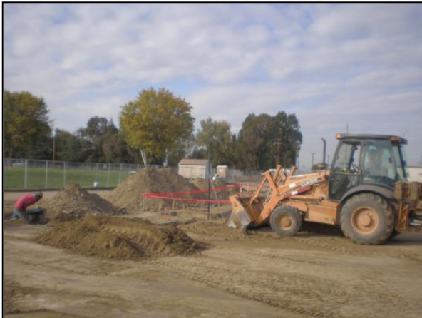
Backfilling Underslab Plumbing Trench
