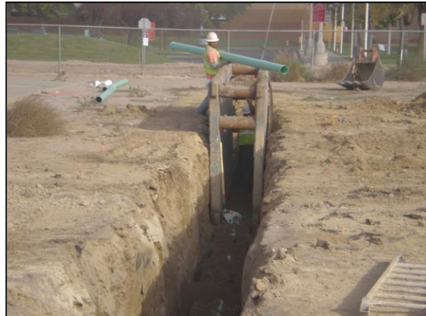
Installing Storm Drain Piping at North End
