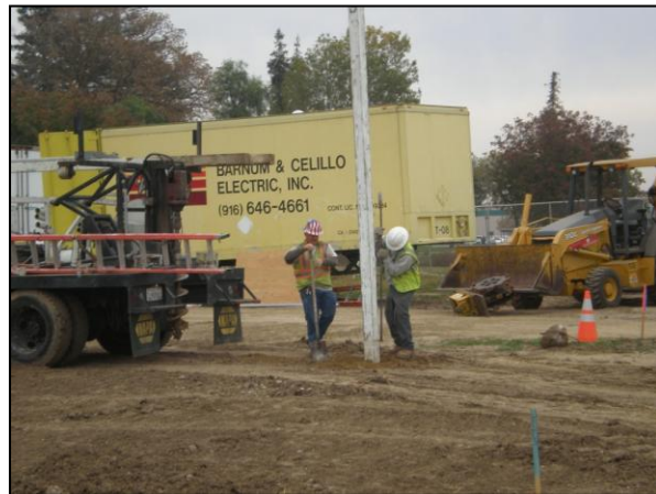
Setting Post for Temporary Electrical Power
