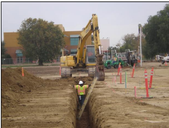
Trenching for Underground Water Piping
