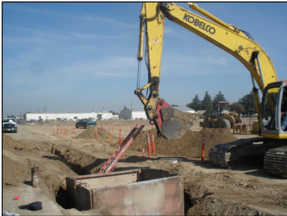
Excavating for Sanitary Sewer System Installation
