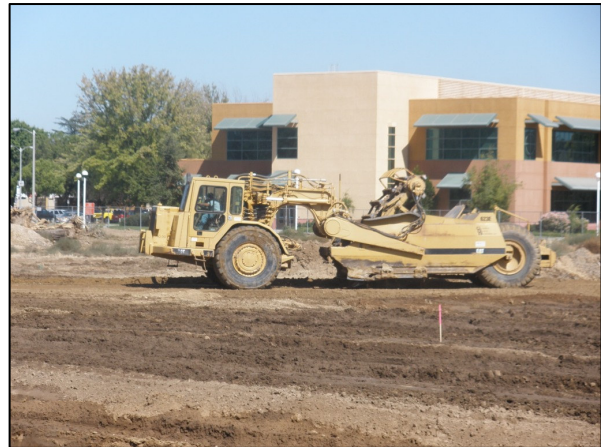
Grading Building Pad
