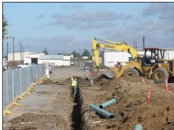
Installing Underground Storm Drain System
