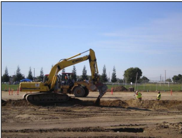
Installing Underground Storm Drain System
