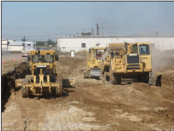
Over-Excavating Building Pad
