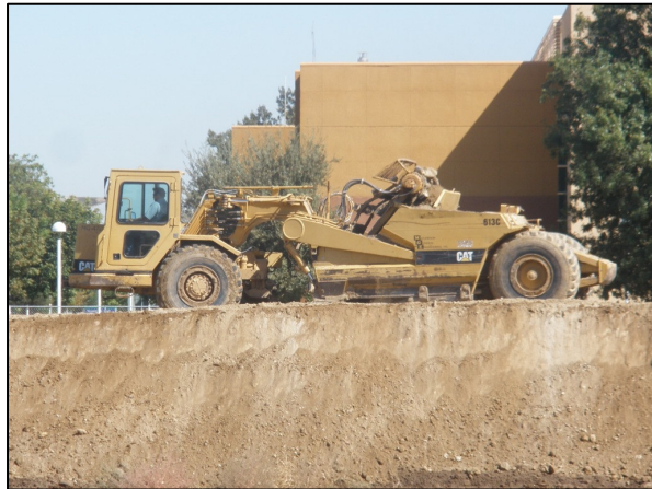
Stock Piling Soil Material
