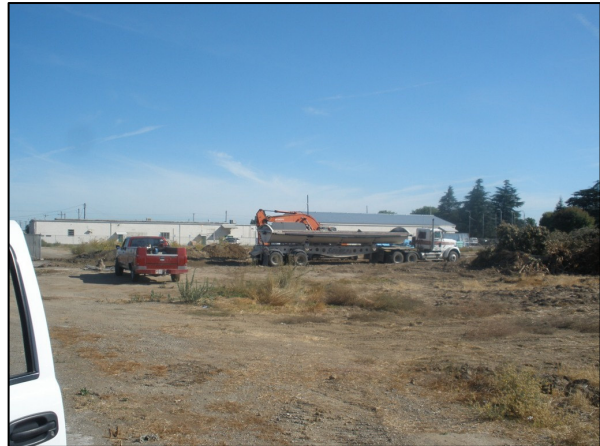
Off Hauling Demolished Asphalt Paving
