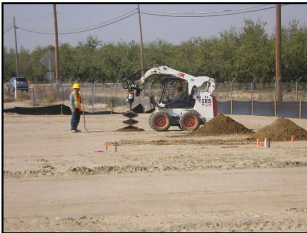
Excavating Column Footings
