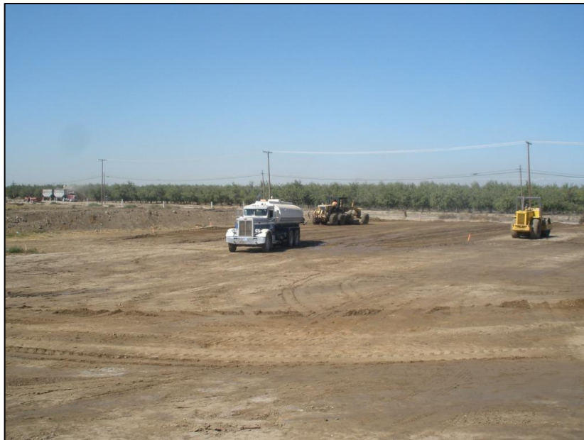
Grading Building Pad
