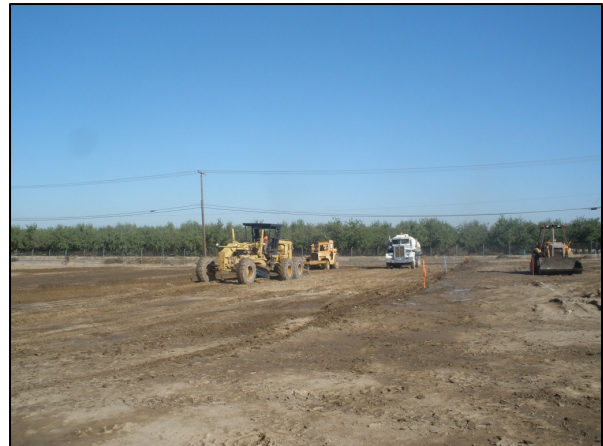
Grading Building Pad
