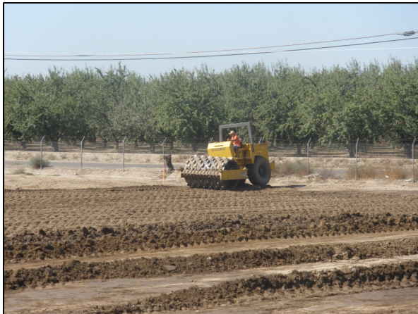
Grading Building Pad
