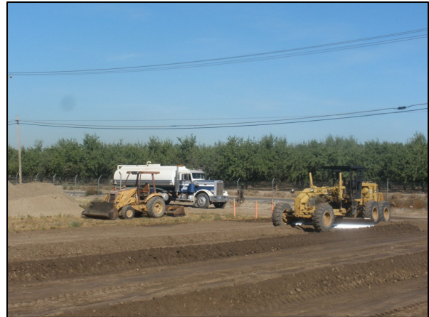
Grading Building Pad
