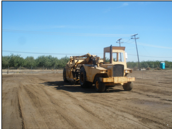
Scraping Soil at Building Pad
