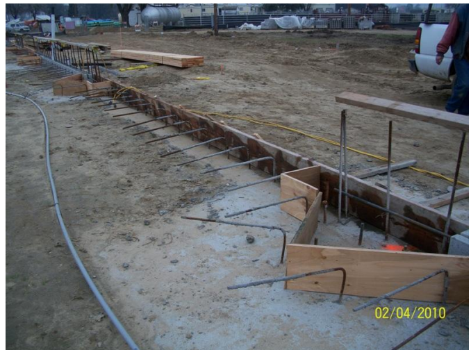
EDGE FORMS FOR SLAB ON GRADE
