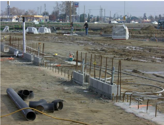
CMU BLOCKS AND UNDERSLAB CONDUITS
