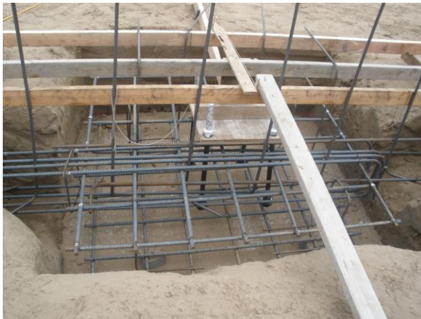
Spread Footing with Anchor Bolt Template
