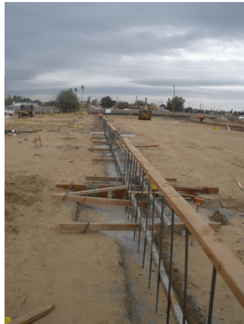
Pouring lean mix at spread footing.
