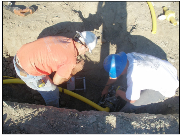
Installing Gas Laterals at Eagle Drive
