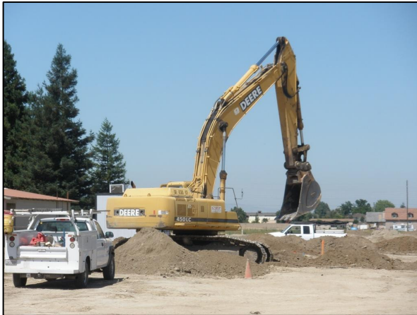
Excavating Water Trench
