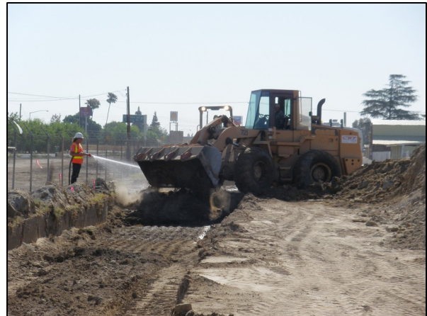
Backfilling Sewer Trench
