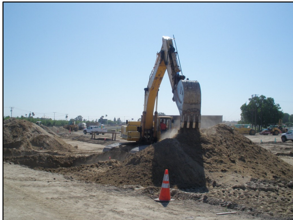
Excavating Sewer Trench
