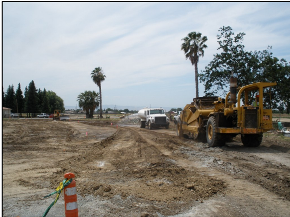
Rough Grading for Building Pads
