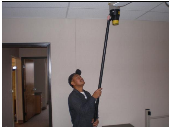
Testing Fire Alarm System
