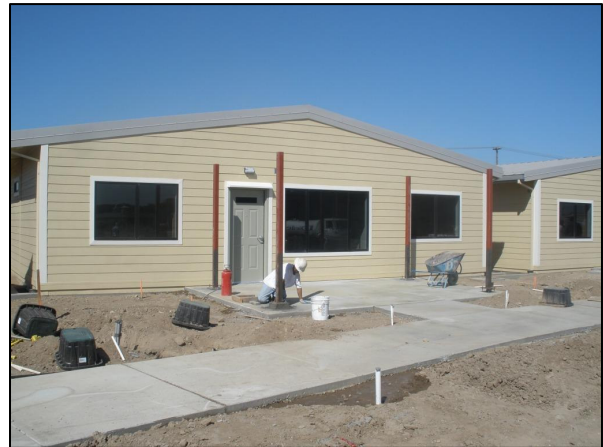
Grouting Column Bases
