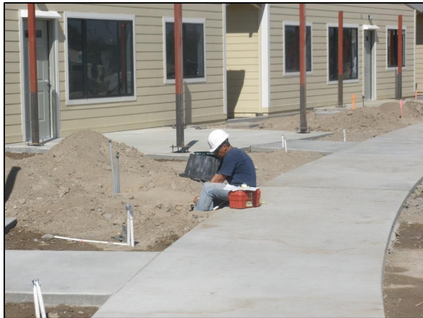
Installing Irrigation Boxes
