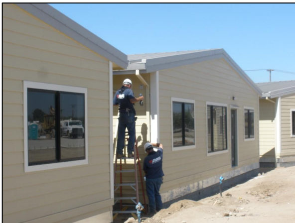
Installing Gutters and Downspouts
