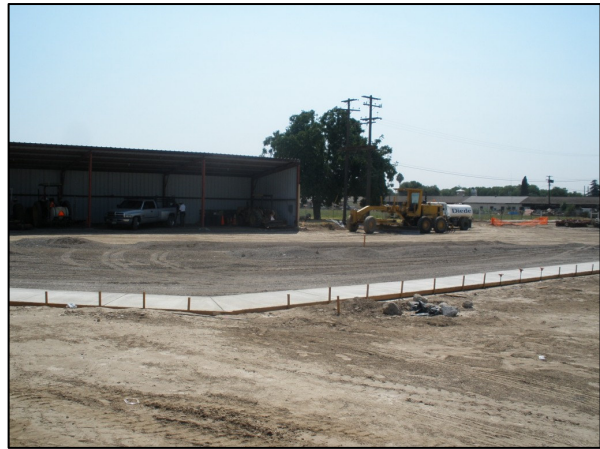
Spreading Base Rock at Fire Truck Access Road
