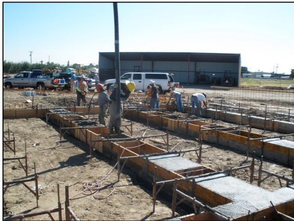
Pouring Building #7 Foundation
