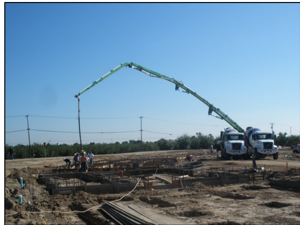
Pouring Building #3 Foundation
