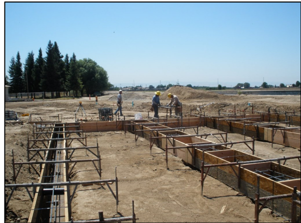
Forming Building 4 Foundation
