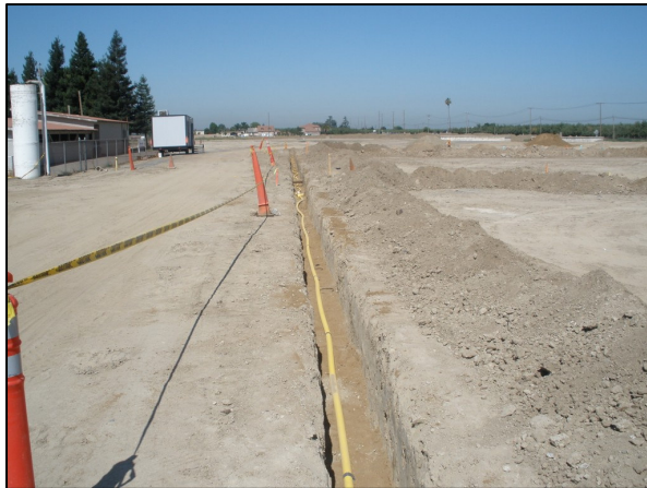
Installing 2" Gas Line
