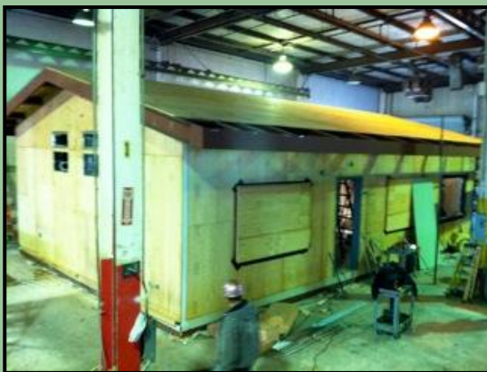
Modular unit under factory construction
