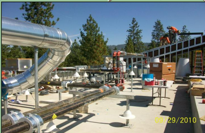
ROOF MECHANICAL AND HYDRONIC PIPING
