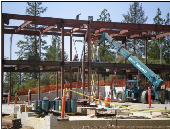
Building steel bracing erection in progress
