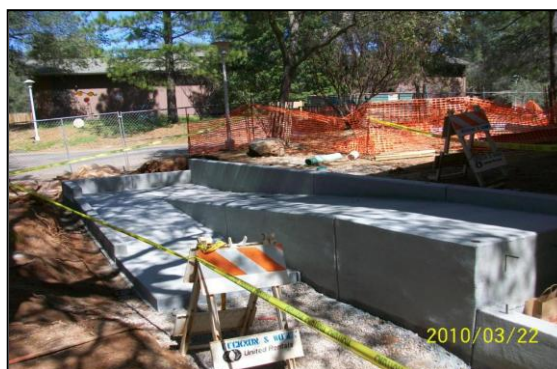
Building "D" disabled ramp installation in progress.
