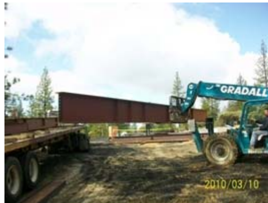
Unloading building steel in progress
