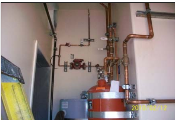
Building E water heater installation in progress
