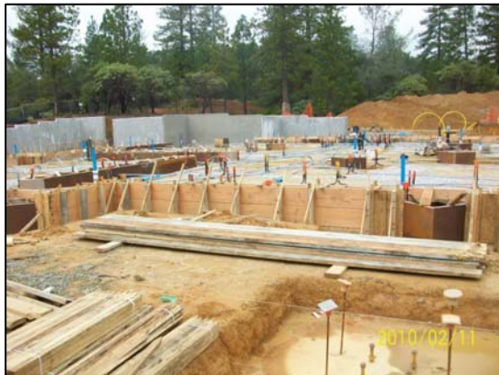
Building slab perimeter forms in progress
