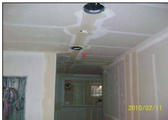
Building "C" drywall installation in progress
