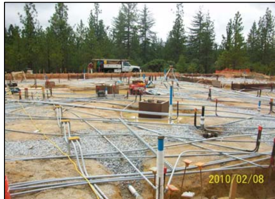
Building under slab electrical and plumbing in progress
