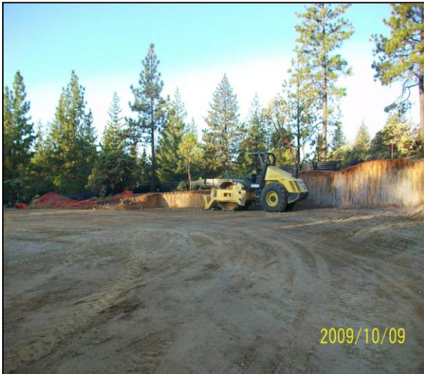
Compacting site for building pad
