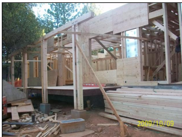
Building "D" wall framing in progress
