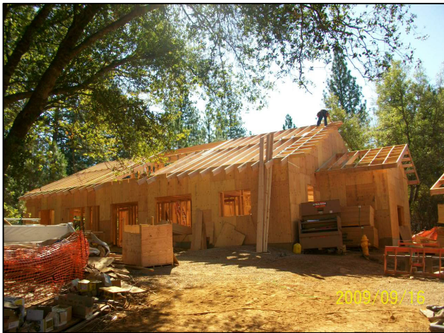
Building "C" roof framing in progress
