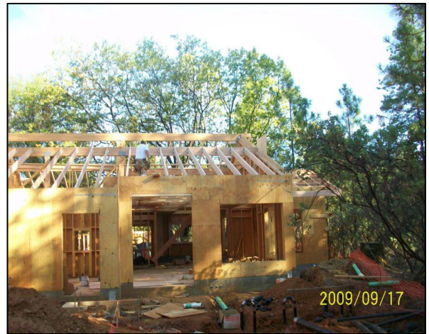
Building "B" roof framing in progress
