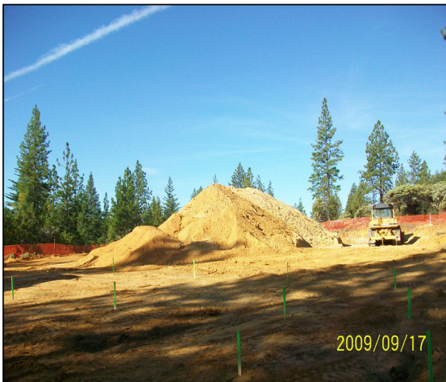
Clearing and excavating site
