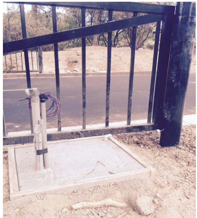
Foundations poured for gate motors
