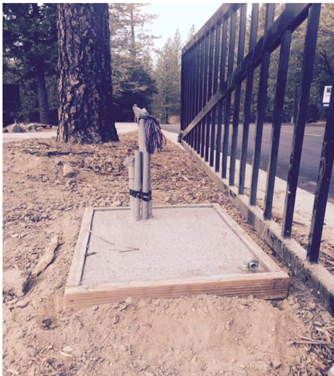
Foundations poured for gate motors
