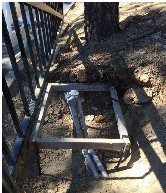
Foundations for motors at gate by Public Safety
