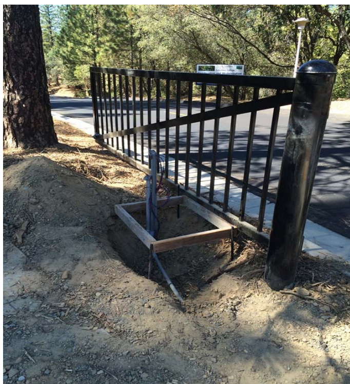
Foundations for motors at gate by Public Safety
