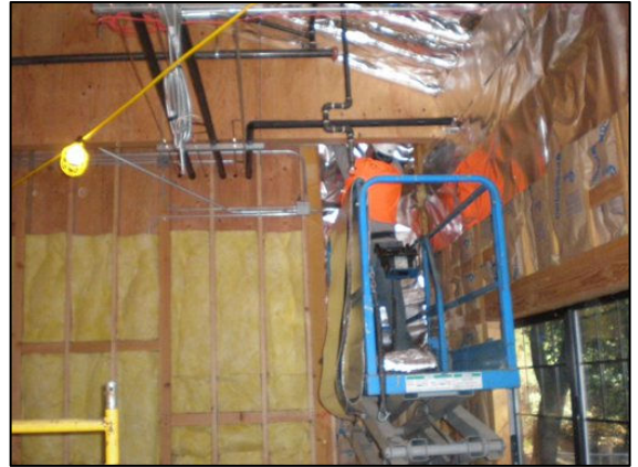
Insulating interior walls
