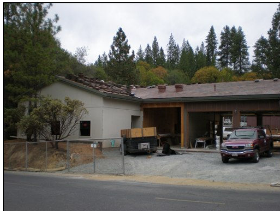
Installing roof tiles
