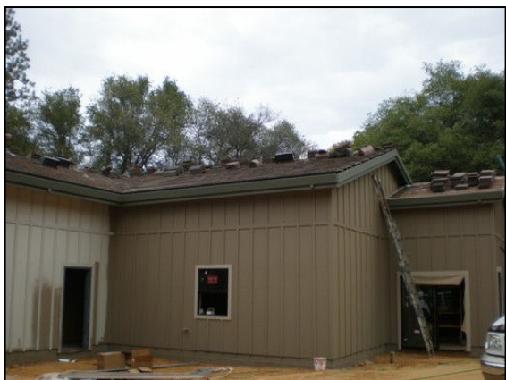
Painting exterior walls & installing roof tiles
