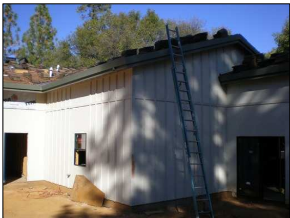
Installing concrete siding & battens
