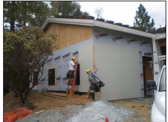
Installing siding
